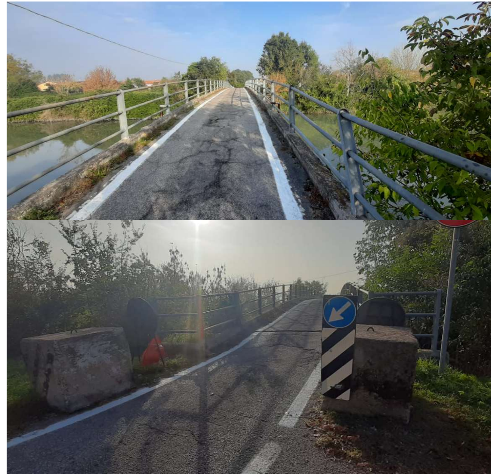
Piano stradale SDF
